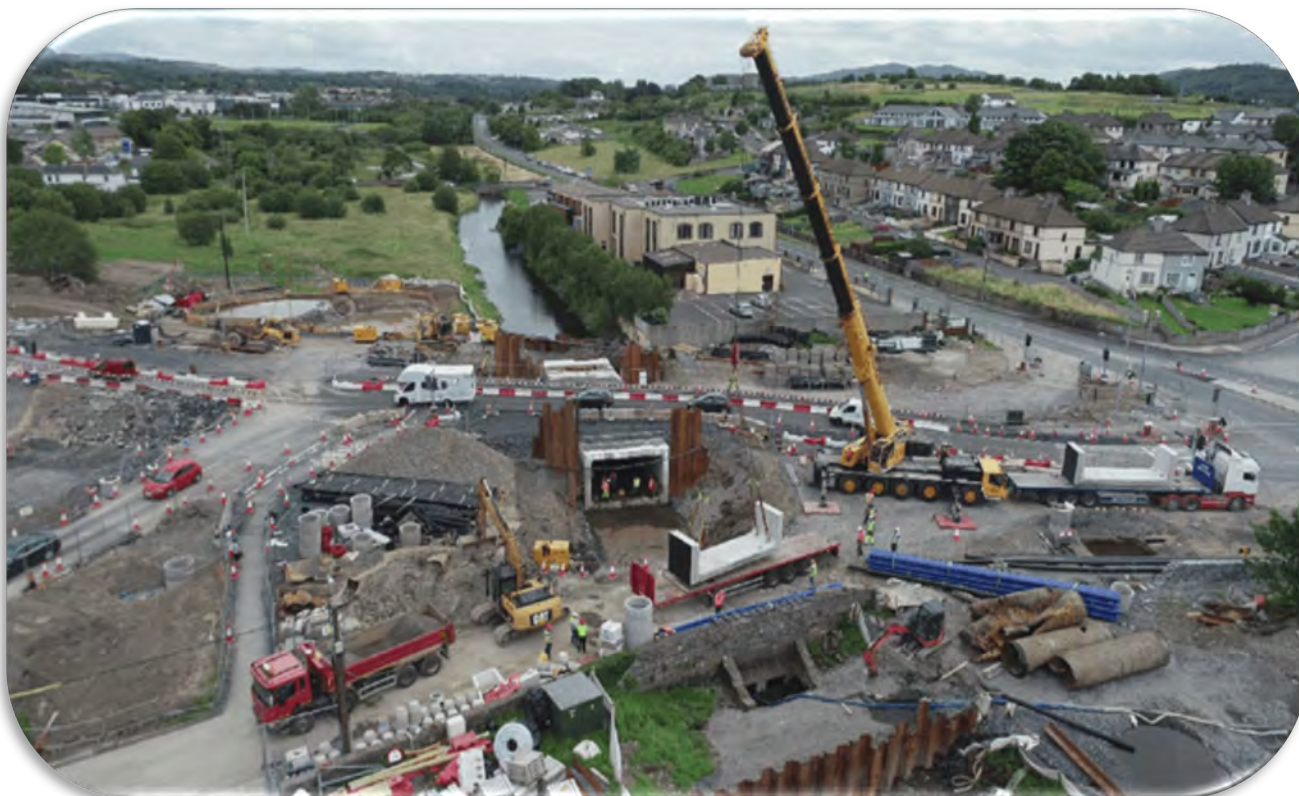
Overview of installation of Copper River Culvert looking east from the outfall at Rosses Point Road Junction - crane lifting in individual precast concrete units
