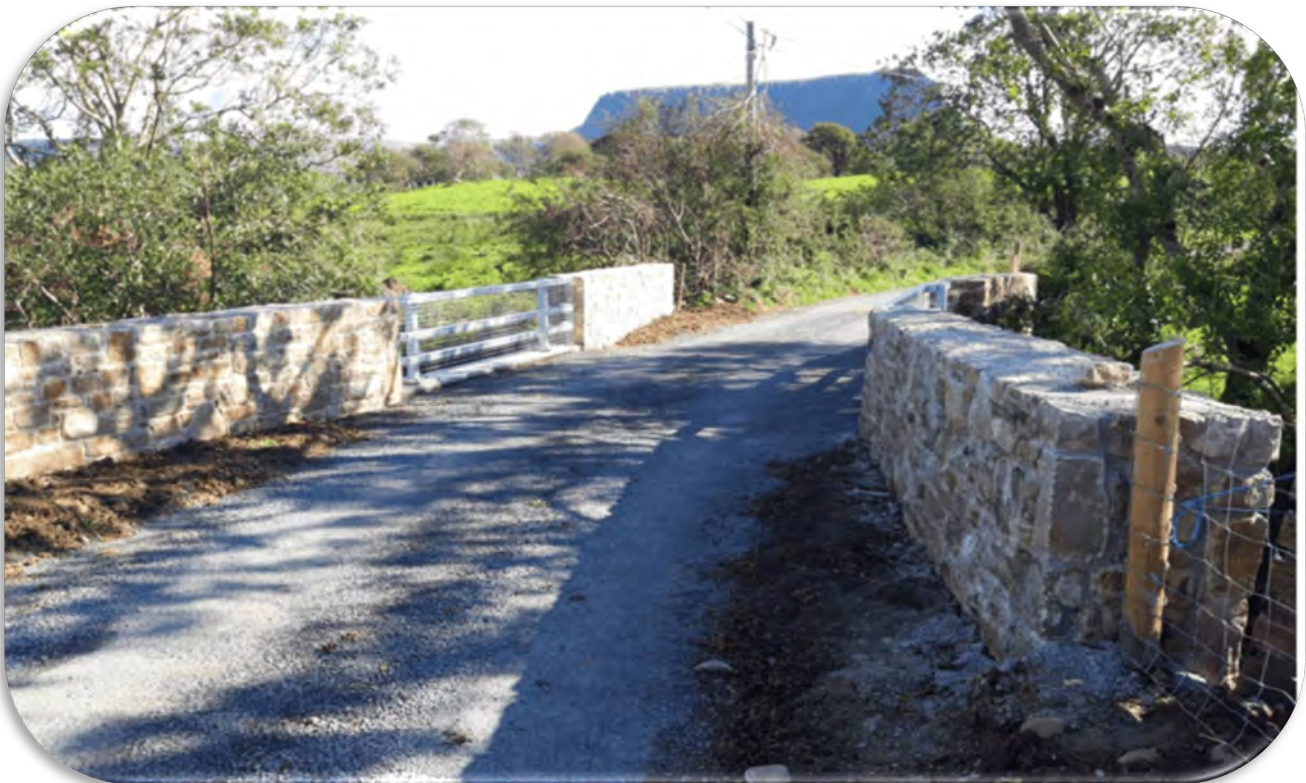
Aghagad Bridge, Grange – new deck, masonry walls and parapet rails
