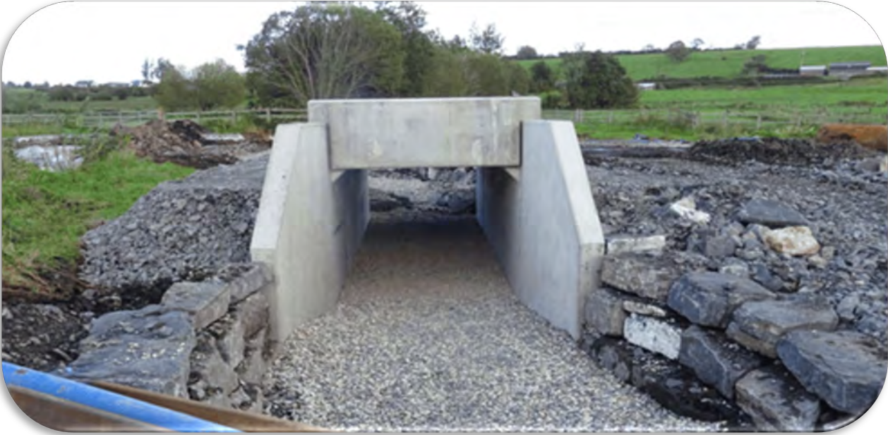
View looking northeast of a culvert under construction in Cloghoge Lower Td. to facilitate a landowner accommodation road (Stream Riverbed mitigation evident)
