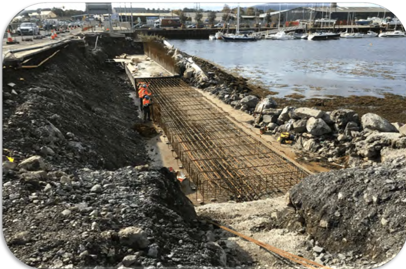
Foundation for Retaining Wall north of Hughes Bridge on Estuary side (west), looking south
