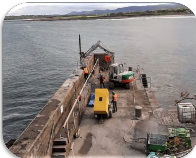
Aughris Pier: Pier head strengthening works - drilling and grouting steel bars down into bedrock
