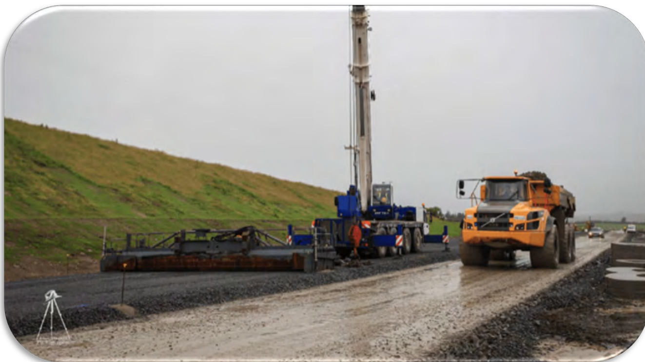
Laying Cement Bound Granular Material (Ch. 10+500)
